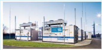
Falkenhagen project (DE) is injecting 2% H 2 by vol. into the gas grid
